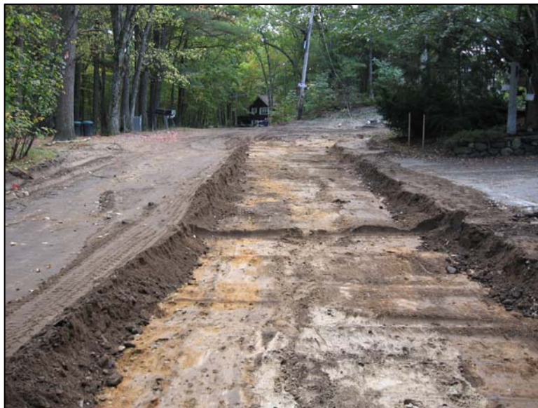
Placement of sub-base material along Shore Drive
