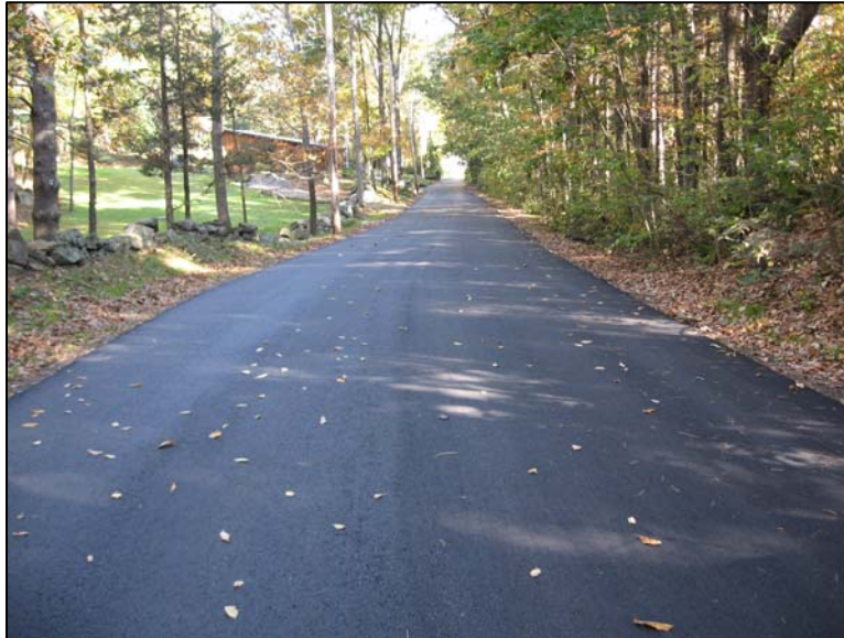
Final wearing course along Wheeler Dam Road
