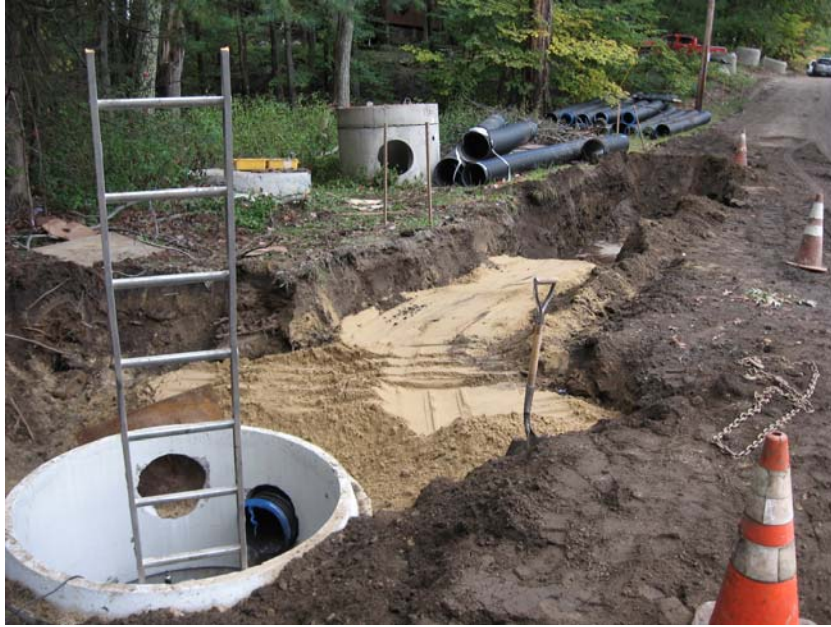
Installation of drainage network along Shore Drive
