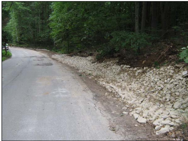
Stone lined swale constructed along Shore Drive
