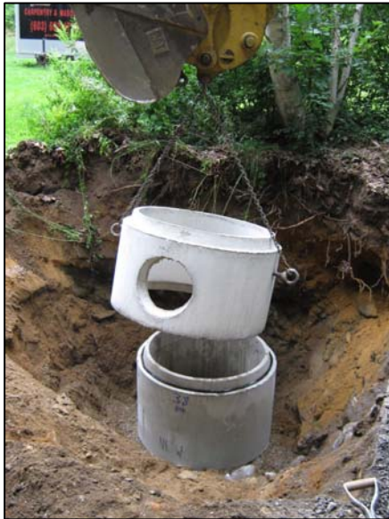
New drainage structure being installed
